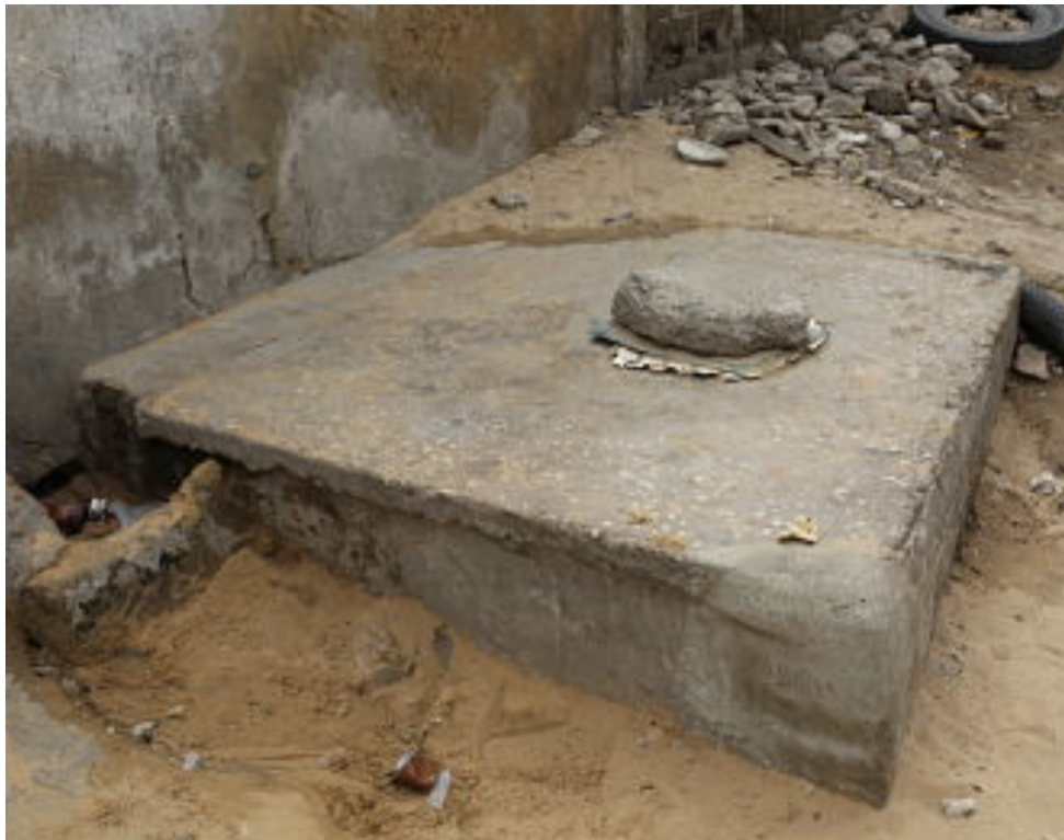
Picture 3 : Septic tank observed in Médina Gounass/Guédiawaye
