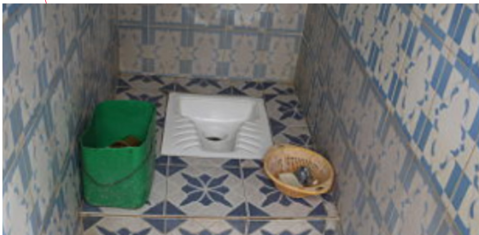
Picture 12 : Clean toilets observed in Golf Sud
