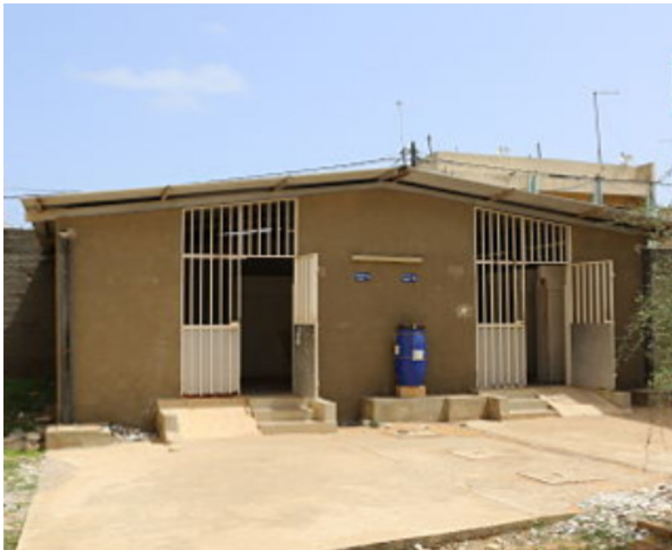
Picture 5 : Separate boys' and girls' toilets with a ramp at CEM APIX/Guinaw rail sud
