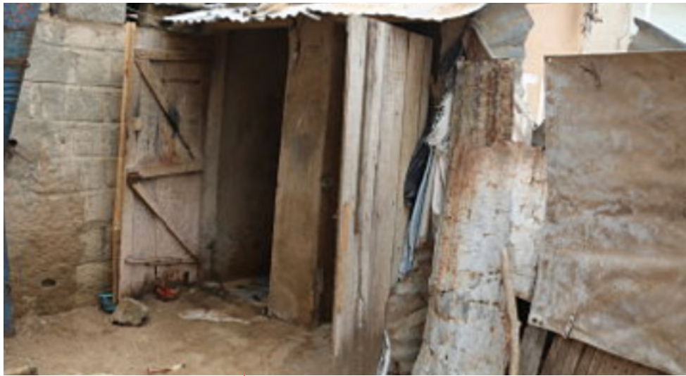
Picture 11 : Dilapidated household toilet observed in Guinaw rail nord
